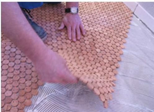
3. Use a water-based contact cement to install the tiles according to manufacturer's instructions. Always follow the Manufacturer's instructions as shown on the adhesive containers. Evenly apply the water based contact cement to both the back of the tile and the substrate. Be sure both surfaces are completely covered. Allow contact cement to fully dry before beginning installation. **Note:** The substrate should be a clean surface, free of any debris.
