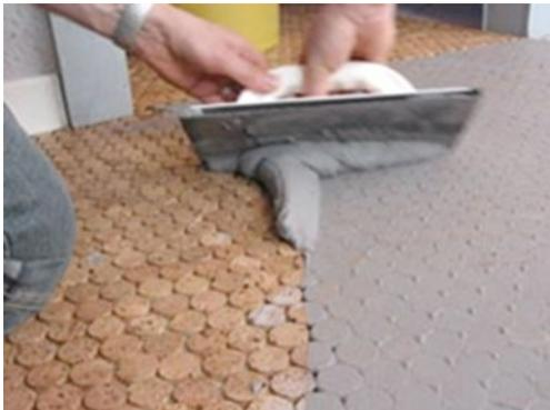
8. Once the water-based polyurethane is dry, evenly distribute the grout (if gap is larger than 1/16" be sure to use sanded grout) with a high quality rubber grout float, making certain all joints are being completely filled to a point level with the top of the cork. The finished joints should be uniformly smooth, without any voids or low spots. **Note:** We recommend using the Cork Mosaic grout supplied by Jelinek Cork.
